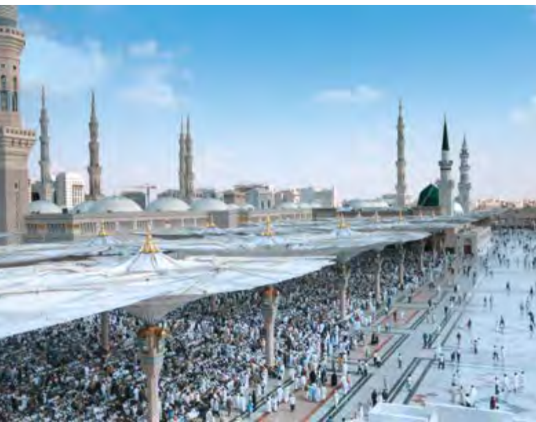
Aussenluftkühlung in Medina, Saudi-Arabien
