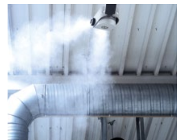
The TurboFog humidifier spray a micro-fine mist as required
